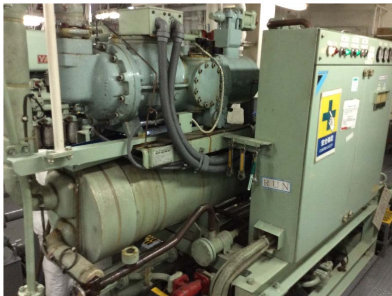
Photograph 2-1-10 Ship's air conditioning system
