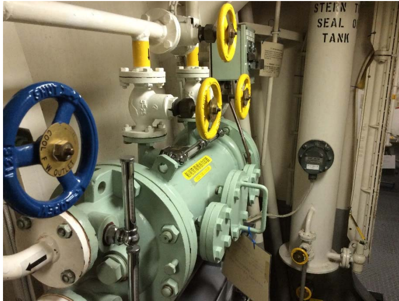
Photo 1-1-1 Seal tank of propeller shaft
