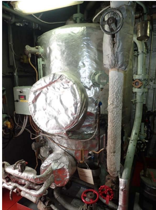
Photo 1-2-3 Waste oil tank
