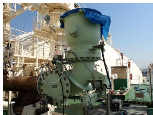
Photo 3: Actually Activated ERS (On-board Equipment) on March 11
